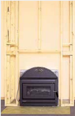
Simple timber frame
